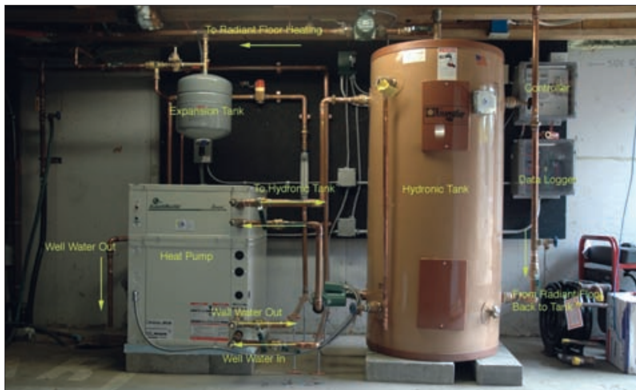
The Genesis unit is connected to an open loop well with a depth of 325 feet, and a recharge rate of 25 GPM; water used for geo-exchange, then discharged into a drain that spills into a wetland nature area. During its first heating season, the system produced about 14.5 million BTUs at an approximate COP of 4.
