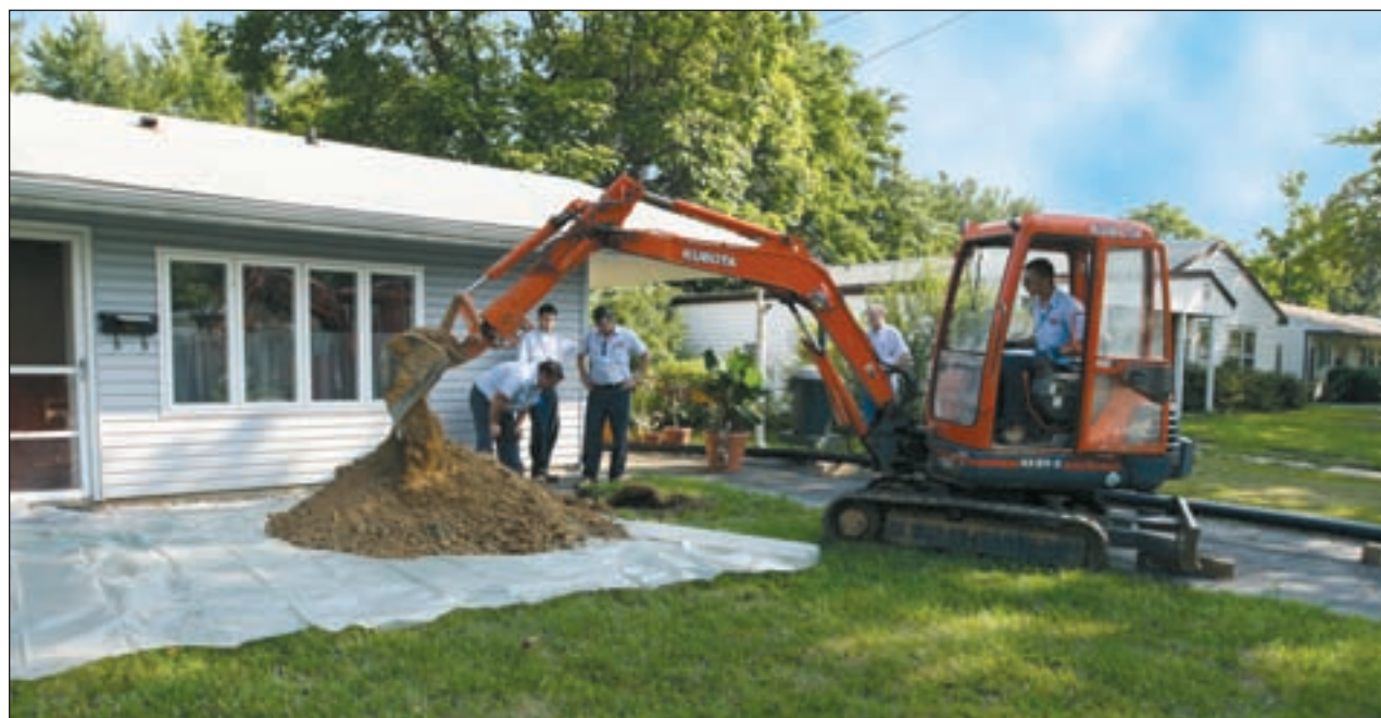
Step 2: Once techs locate the trouble spots, they dig small access points so they can reach the sewer line. With this advanced "trenchless" technology, they no longer have to dig up entire yards, costly landscaping or pavement.
