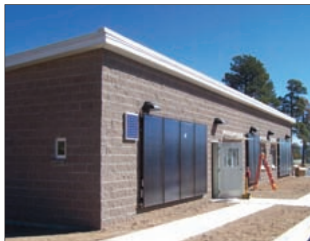
Flat plate solar collectors on a vertical wall are filled with a 50% mixture of non-toxic, high-temperature-inhibited propylene glycol and 50% water, circulated by a direct current pump, powered by a 30-watt photovoltaic (PV) module. South face of Eco Station uses PV panel for solar glycol pump (30-watt rating) and Viessmann solar heat collectors with shipping covers removed.
