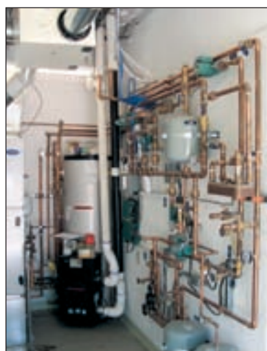
Hydronic heating system in mechanical room. Components include: Voyager 80-gallon stainless steel storage tank with condensing boiler gas back up for heat and domestic hot water; Taco circulating pumps (green pumps); Crown "brazed plate" heat exchanger CBP5X12-20 (foreground right); Laing PV-direct solar glycol circulator (small bronze and black/silver pump); Taco EBV zone valves (near the floor); ZVC control boxes and SR relay enclosures (green boxes); and Tekmar 155 and 152 differential and set-point controls (mounted on gray box).
