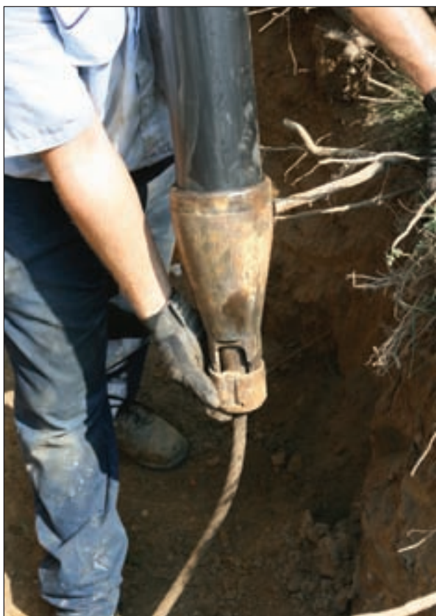
Step 3: A cable is inserted into the faulty pipeline; and Step 4: The cable is pulled through the path of the existing line. It bursts the old pipe, simultaneously pulling the replacement line into position.
