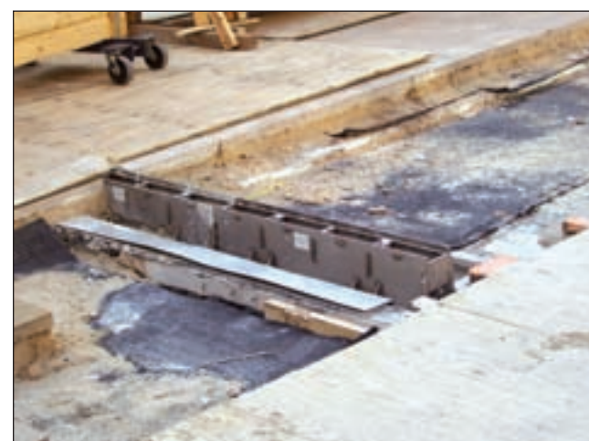
Jay R. Smith Mfg. Co., working from the architectural drawings, created four different custom fabricated stainless steel trench drains, designed to specifically adapt and install around existing building structures. The drains add an appeal to an otherwise unnoticeable application: "All of the stainless steel trench drain designs gave us functionality and visual appeal," says David Glick of FX Fowle Architects.
