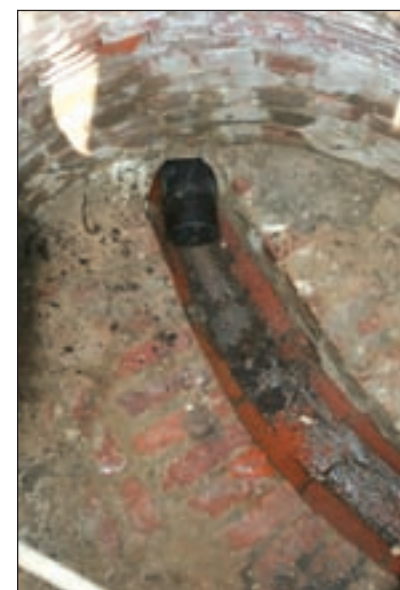
Step 5. The old pipe disintegrates. The new polyurethane pipe lasts as long as 50 years.
