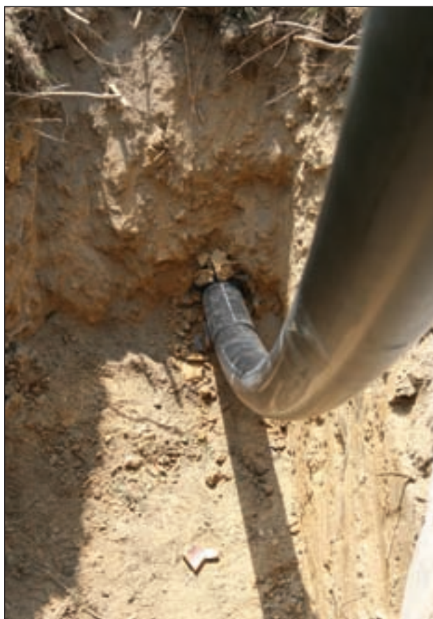
Step 3: A cable is inserted into the faulty pipeline; and Step 4: The cable is pulled through the path of the existing line. It bursts the old pipe, simultaneously pulling the replacement line into position.
