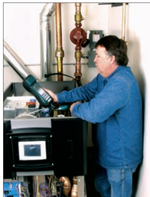
Pat Noonan, VP and part owner of Par Mechanical, Montrose, Colo., installs diagnostic instrumentation specified by Laars to monitor the boiler's high altitude operation.
