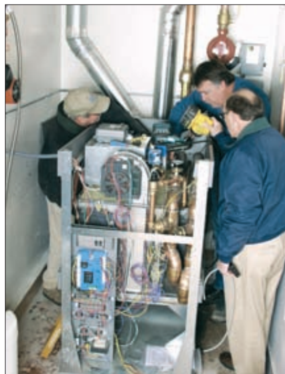
A crew installed the 1 million BTU MagnaTherm a few days before Christmas 2009, also running copper lines to several fan coil units in the 10,000-sq.-ft. gymnasium.
