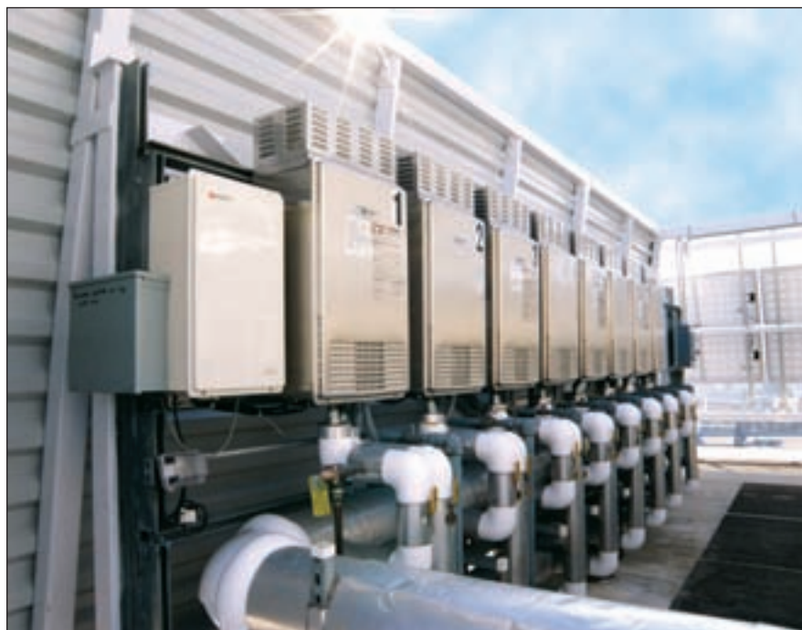
Eight Noritz N-1321M-ASME commercial water heaters on the rooftop supply hot water for the soak tubs in the hotel’s 208 guest rooms.
