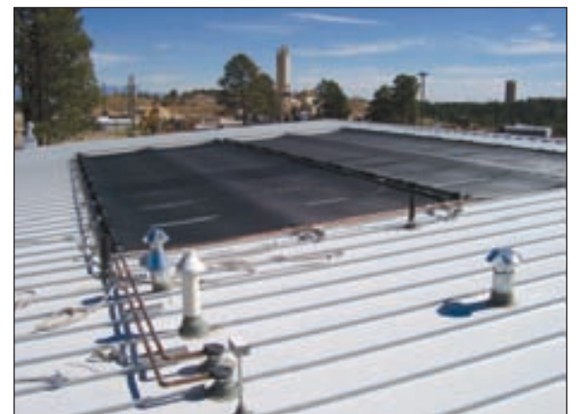
Un glazed solar heat exchanger panels mounted horizontally on the roof help provide summer cooling in the building via night sky radiant cooling. Heat is removed from the mass floors by circulating boiler fluid through the floors at night, passing this heat “backward” through the panels, where it is cooled by radiation to the night sky. Roof of Eco Station features Heliocol HC-50 un glazed plastic radiator panels for cooling.
