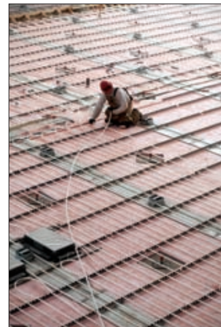
Maximum capacity of a radiant floor cooling system is about 14 Btu per hour per square foot when using a design set-point temperature of 78°F.
