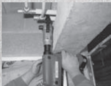
THE P20+ CORDLESS PRESSING TOOL FOR 1" TO 4" TUBING
