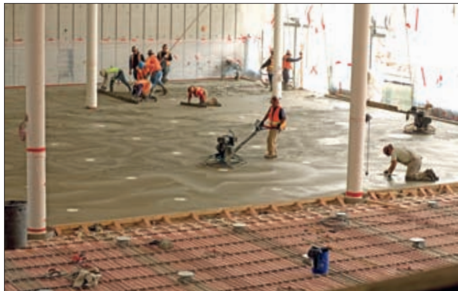
High-mass radiant cooling uses tubing embedded in the concrete floor and/or walls and is common in hybrid systems that both cool and heat a structure.
