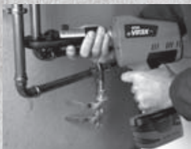
THE M20+ CORDLESS PRESSING TOOL FOR 1/2" TO 1" COPPER TUBING
