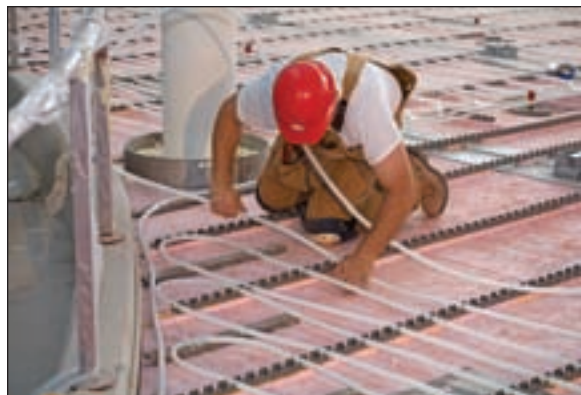
Radiant cooling systems work like radiant heat in reverse, circulating chilled water or water-glycol fluid through tubing embedded in the structure.
