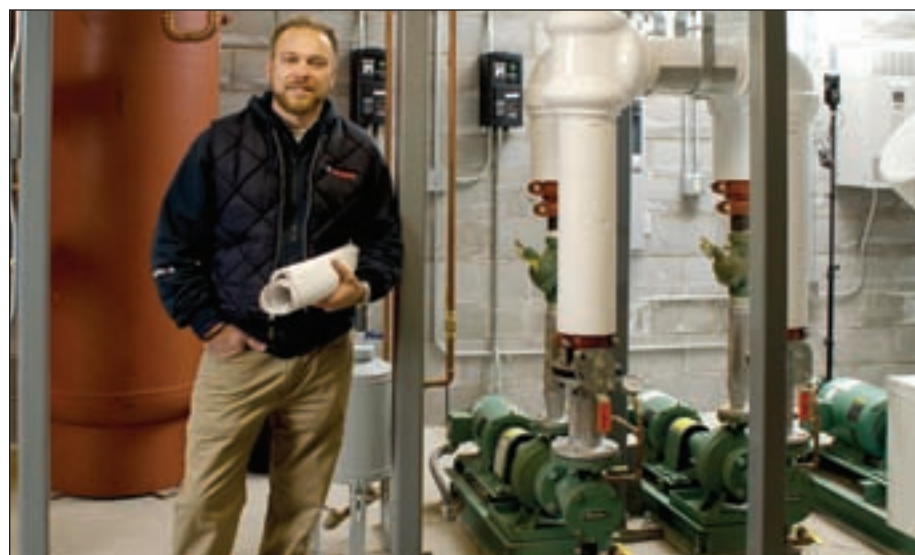
Drew Nowak, MJ Mechanical's design-project coordinator proposed Taco's single pipe LoadMatch system for the Maxim Medical Center project. LoadMatch requires less pipe, eliminates control valves and reduces balancing valves to a minimum.
