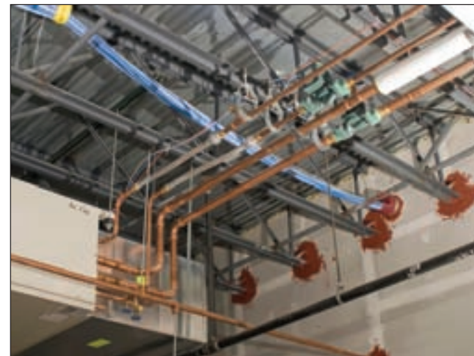
Nowak then finalized the design, employing just over 100 LoadMatch circulators and McQuay fan coils, and added a thermal ice storage system to save additional energy.
