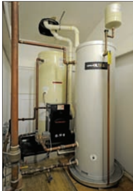
Voyager stainless steel water heater, with an input of 199,000 Btu/h and 45 gallons of internal storage (background), is coupled with an 80-gallon SuperStor Ultra storage tank (foreground) to provide hot water to 16 guest rooms.
