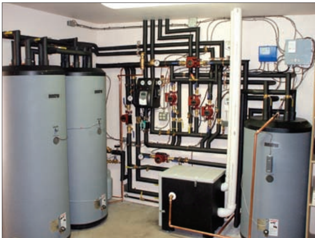
Sky Farm’s Oventrop solar radiant and domestic hot water system utilizes five evacuated tube solar collectors (top), and (below) one 80-gallon dual-coil stainless steel indirect domestic hot water solar storage tank; two 115-gallon single-coil stainless steel solar storage tanks; and a Regusol EL130 solar pumping and control station. The solar closed loop system is designed with an Oventrop Pro dual pump logic controller, which prioritizes solar domestic hot water production.
