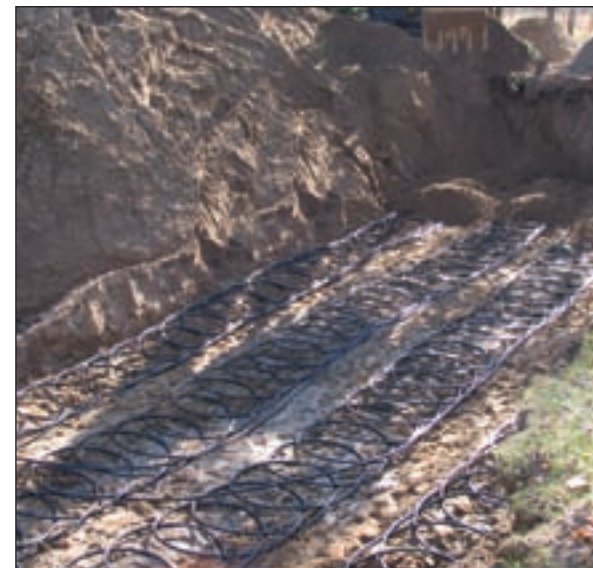
Similar to the image above, the loops of tubing that go underground are the heart of the nature center's geothermal heat transfer system.
