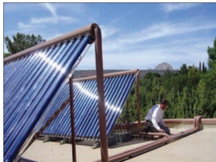
Sky Farm’s Oventrop solar radiant and domestic hot water system utilizes five evacuated tube solar collectors (top), and (below) one 80-gallon dual-coil stainless steel indirect domestic hot water solar storage tank; two 115-gallon single-coil stainless steel solar storage tanks; and a Regusol EL130 solar pumping and control station. The solar closed loop system is designed with an Oventrop Pro dual pump logic controller, which prioritizes solar domestic hot water production.
