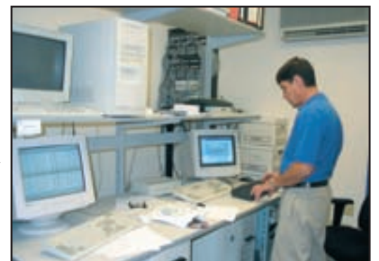
President Ronnie Cosentino in the computer room that houses servers and equipment.
