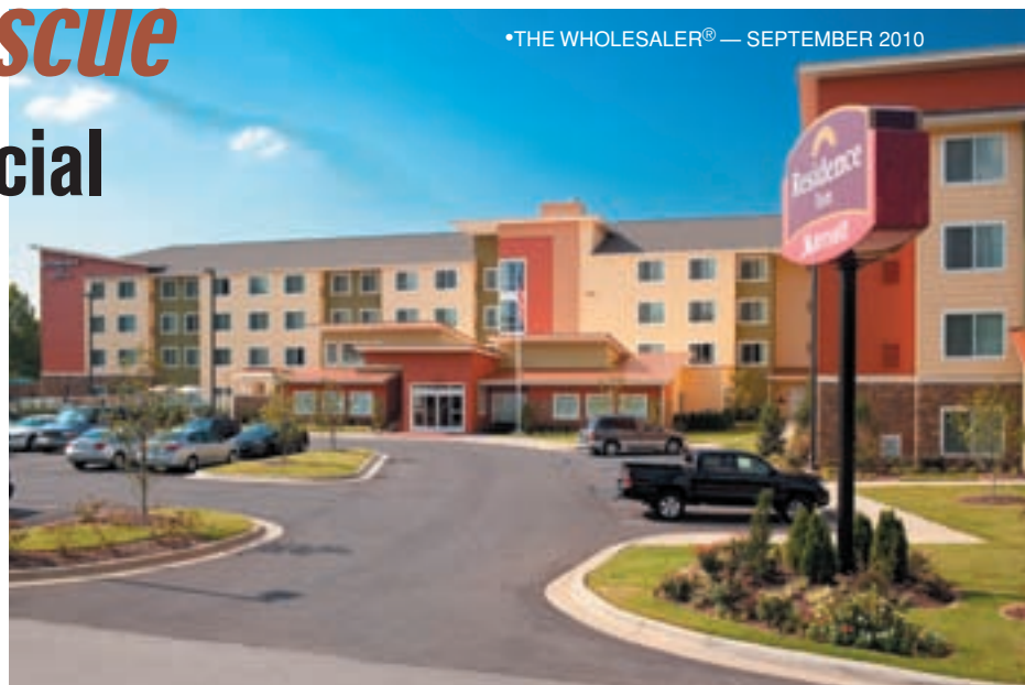
At The Residence Inn in Florence, Ala., the tankless water heating and common venting solutions proved so effective that the hotel owner anticipates going with this approach on future hotel projects.
