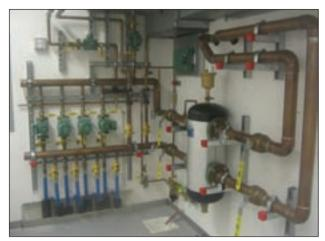
The 2-inch Calleffi Hydraulic separator provides the central organization for this elegantly constructed mechanical space. This mechanical room can be easily understood and serviced. Photo courtesy Mayo Mechanical.
