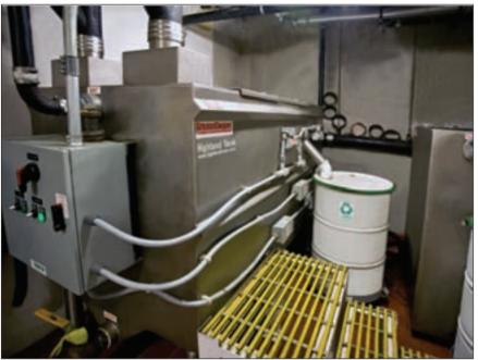
Highland Tank worked with the engineers on a job for a large supermarket chain in New York City. They provided a solution to avoid the cost of multiple grease interceptors and instead install one large automatic grease interceptor.
