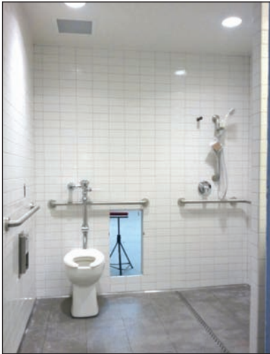
Fig. 3: Interior of a nearly finished PIVOTek hospital pod. Note the trench style shower drain specific to this installation.
