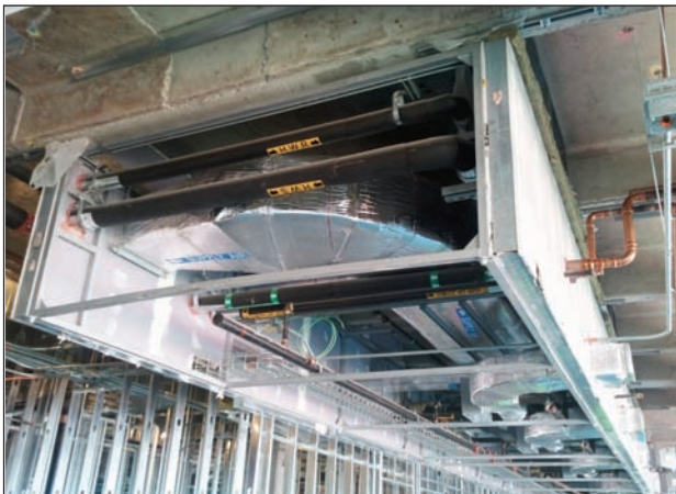
Fig. 1: Corridor ceiling module. Note that corridor studs have been installed on the left side of the corridor but not yet on the right.
