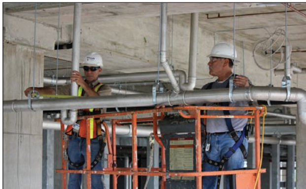
One of the most unique facets of the new facility's construction was the specification for 8,000 lineal feet of stainless steel drainage piping
