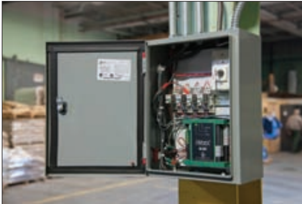
A single LCI (local control interface) controls all the units from one on-site location.
