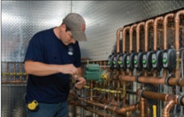
In this photo, variable speed circulators are used in conjunction with zone valves.
