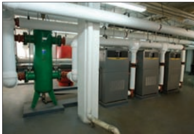
Condensing boilers, like the Rheos+ or NeoTherm boilers, are built to extract latent heat from the moisture that forms in the condensing heat exchanger, dramatically enhancing combustion efficiency.”
