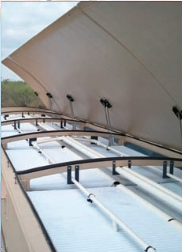
AdvanTex® AXMAX Treatment System utilizing textile filter media and micro-dosing spray nozzles. Photo courtesy of Orenco Systems®, Inc.
