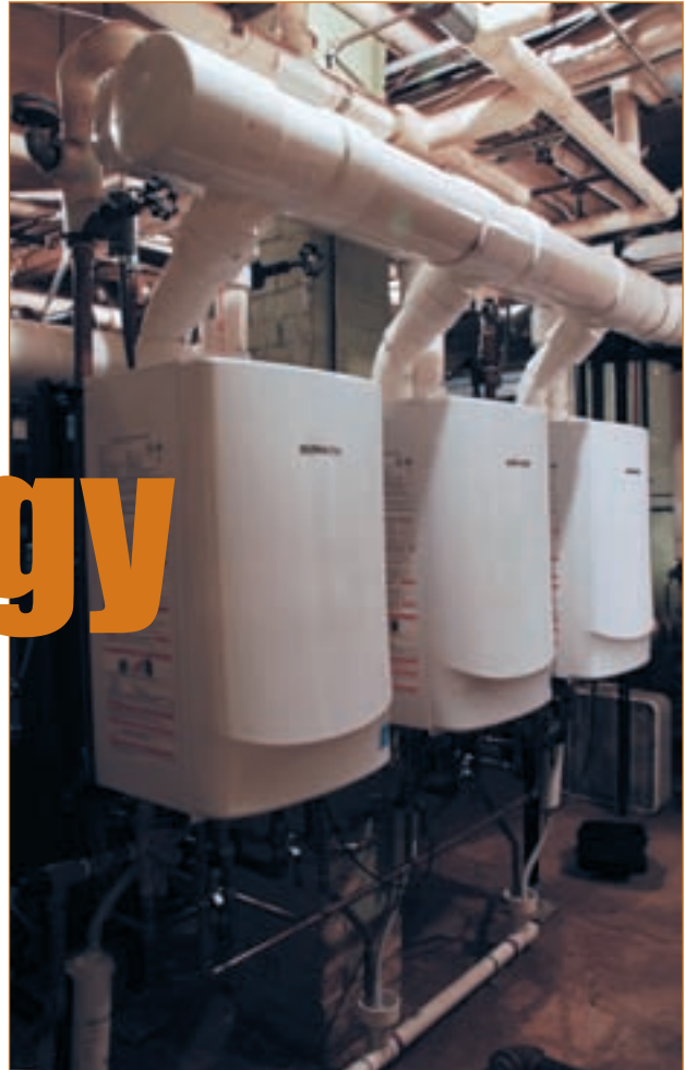
Metropolitan Industries replaced the old tank water heaters with three Navien NR240A natural gas tankless water heaters, each rated 98% efficient with a Btu rating of 199,000, drastically reducing the cost of heating the mansion's water.
