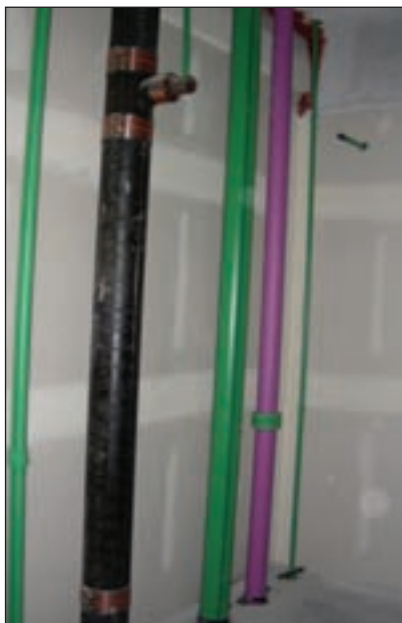
Aquatherm's Lilac piping is colored to differentiate potable water use.
