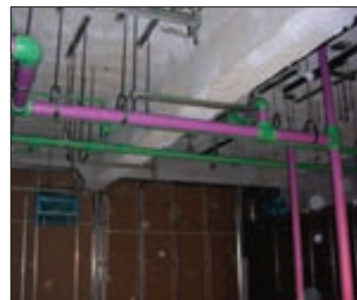
Rainwater is used in the reclaimed system, with Aquatherm's Lilac piping transporting it to low-flow toilets and urinals.
