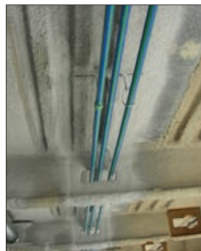
McKinstry utilized Aquatherm's 1/2-in.-diameter Greenpipe® pressure piping.
