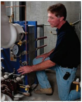
Tim Mayer checks the amount of pressure drop through a plate and frame heat exchanger.
