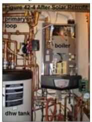
installation would have been much more difficult and much less serviceable without the ceiling mounted primary loop.
