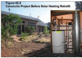
The only heating fuel available is propane, and the original gas burner was a Lochinvar DDL075 that provided both potable DHW and boiler fluid for the floors (seen on the right in Fig.42-2). This resembles a conventional 75gallon gas water heater tank, but has a heat exchanger coil
